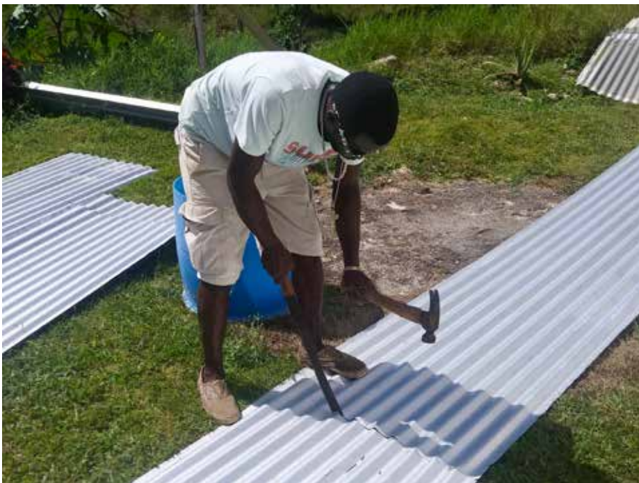
Cutting roof panels with a machete
