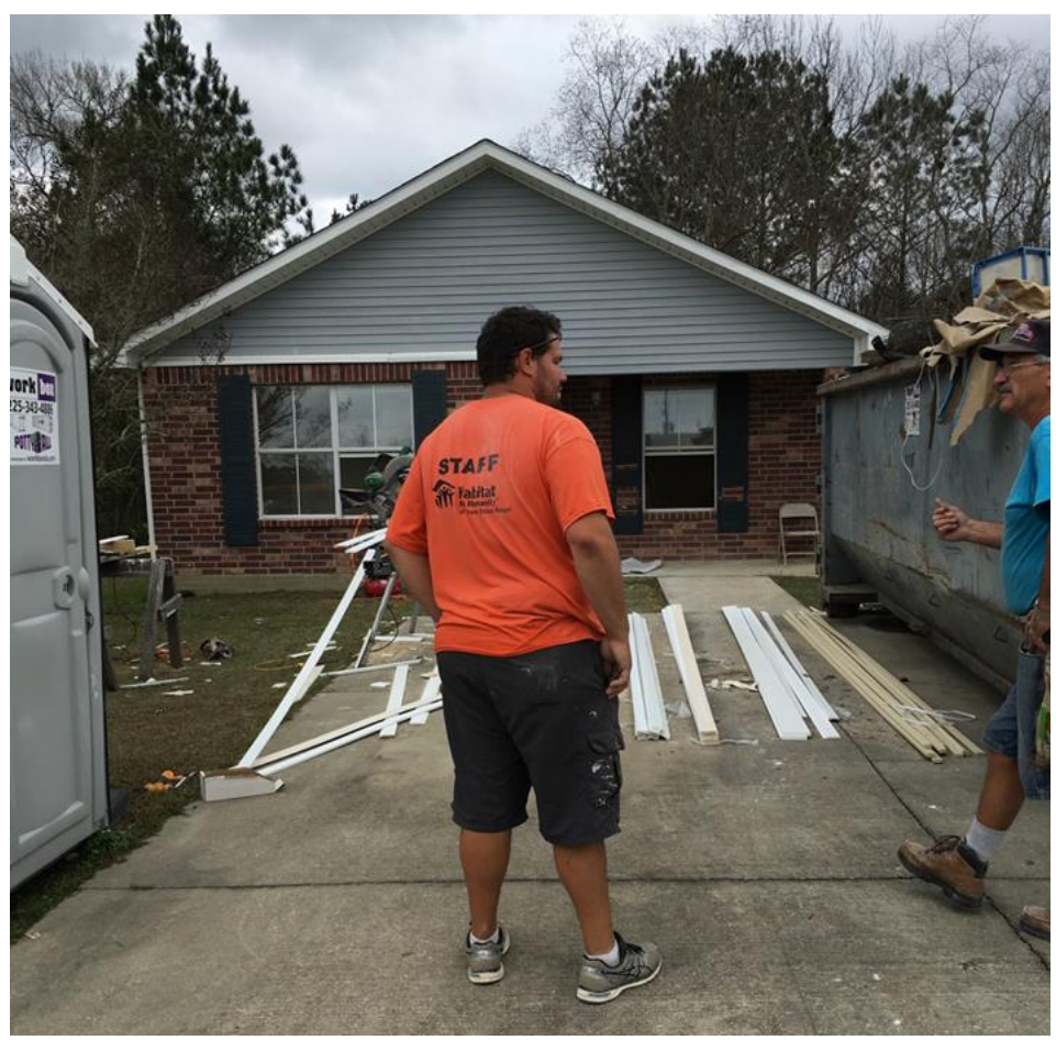
Volunteers working on replacing trim inside damaged home
