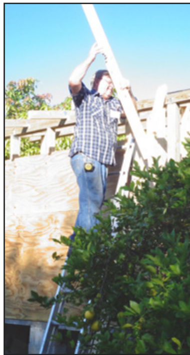
↑ Hank Huigenbos, Wingham, ON, rebuilding one of the demonstration buildings that were destroyed by the hurricane.
