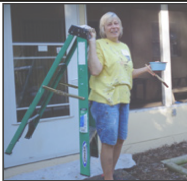
↑ After the hurricane lots of buildings needed pressure washing and painting. Lynn Ballard, Remsen, NY working on one of the seven buildings that were painted.
