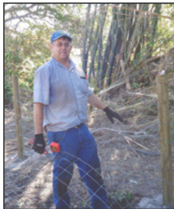
↑ Ron Herrold, IN repairing the perimeter fence at ECHO. Hurricane Irma blew down many trees on the property in Ft. Myers, FL destroying the fence.
