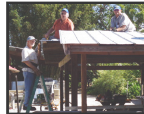
↑ Robert Morton, NY, Melvin Bell, IL and Ron Herrold, IN repairing a roof after the hurricane.
