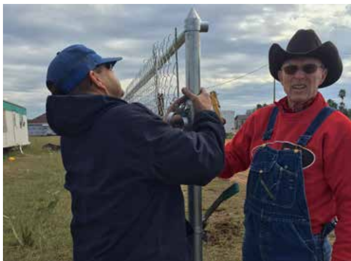
Monday morning, the work began with Andy Dahlquist, Dave Ferris, Bob Hibma, and Ron Herrold starting a perimeter fence around the lot and work site.
