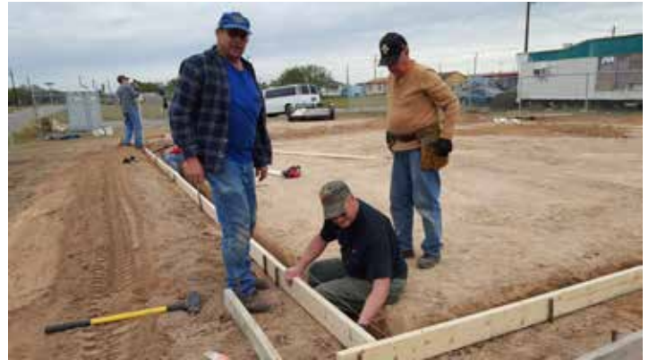
Then Richard Binder brought the back hoe and began the dirt work, removing a few inches of top soil and putting a foot of sand on which to pour the concrete. After forming and putting in the plumbing, they hired a cement crew to pour the pad. They did a great job (with Richard's help).
