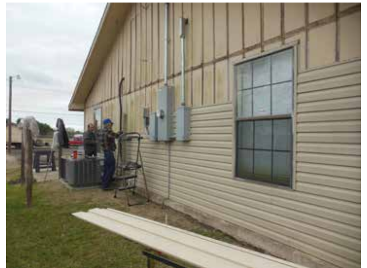
Meanwhile, Bert Henriksen, Bruce Burton, Ernie Laird, Karen Binder, and Deb Herrold removed old, rotten boards and installed new vinyl siding on Emmanuel Baptist Church, north of Edinburg.
